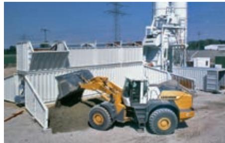
Backfilling of the ramps to the in-line silo compartments
