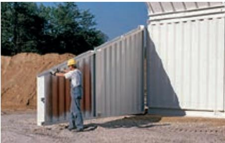
Unfolding the sheet pilings at the in-line silo
