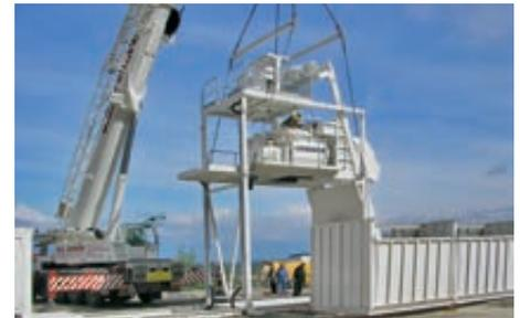
Fixation of the Mobilmix in unfolded state
