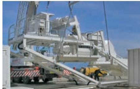
Unfolding the Mobilmix mounted on steel foundations
